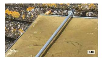
Slide the two locking bars through the four locating holes in the tray above the slabs and secure using a cotter pin through the eyelet in the end of the locking bar.
