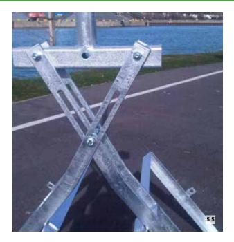
5.9 Once in position ensure that the two trays both sit flat against the roof sheet before tightening the nuts and bolts that secure the T-bar to the arms and the arms to each other, checking at all times that the centre pole remains vertical during the tightening process, tighten all 4 pairs of nuts and bolts to 50Nm.
